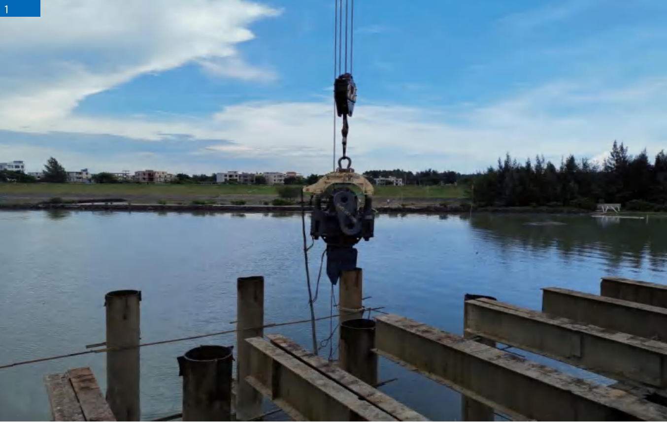
DZJ-400 2 港珠澳大桥 Hong Kong-Zhuhai-Macao Bridge 使用单位：中铁大桥局 User: China Railway Major Bridge Engineering 施工情况：围堰拼桩拆除，及海上风电桩打入 Construction situation: Extract cofferdam piles and piling offshore wind power piles 地质情况：淤泥，红土，石灰岩 Geological conditions: Silty clay with silt
