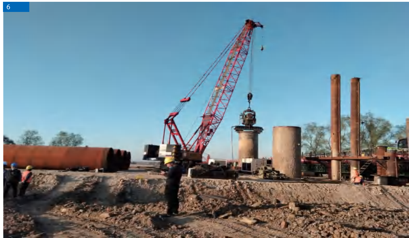
DZJ-135 4 洪湾旧村改造工程 Hongwan Old Village Reconstruction Project 施工情况：桩径8.3m，桩长36m，管桩壁厚12mm Construction situation: 8.3m diameter,36m long and wall thickness 12mm steel pipe pile 入土深度：24m Depth of penetration: 24m 地质情况：淤泥层，细沙粘土层，全风化花岗岩层 Geological conditions: Silt layer,sand clay layer, fully weathered granite layer
