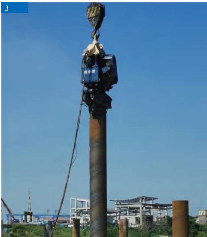
DZJ-400 2 港珠澳大桥 Hong Kong-Zhuhai-Macao Bridge 使用单位：中铁大桥局 User: China Railway Major Bridge Engineering 施工情况：围堰拼桩拆除，及海上风电桩打入 Construction situation: Extract cofferdam piles and piling offshore wind power piles 地质情况：淤泥，红土，石灰岩 Geological conditions: Silty clay with silt
