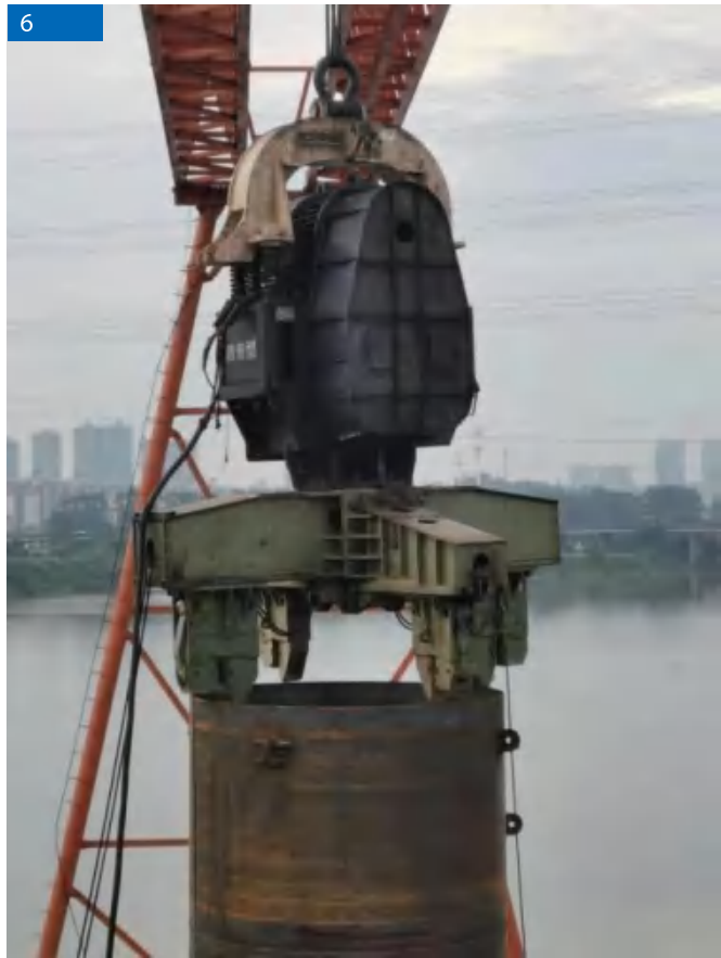
DZJ -90 4 银川吴银客运铁路 Yinchuan Wuyin Passenger railway 施工情况：管桩18m，直径800 Construction situation: 800mm diameter and 18m long pipe pile 地质情况：沙土鹅软石 Geological conditions: Sand cobblestone
