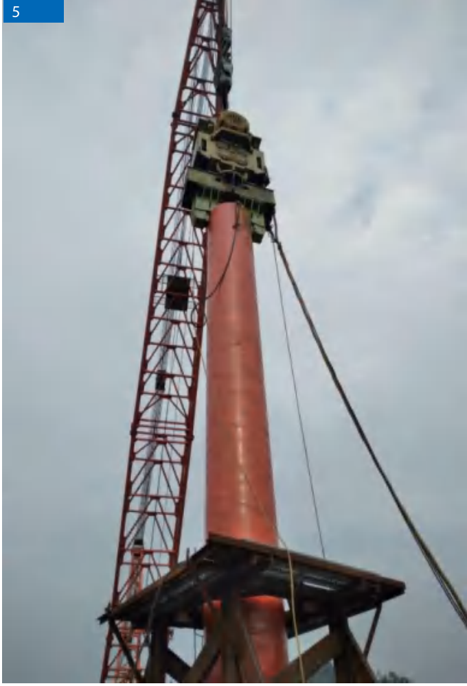
DZJ -90 4 银川吴银客运铁路 Yinchuan Wuyin Passenger railway 施工情况：管桩18m，直径800 Construction situation: 800mm diameter and 18m long pipe pile 地质情况：沙土鹅软石 Geological conditions: Sand cobblestone
