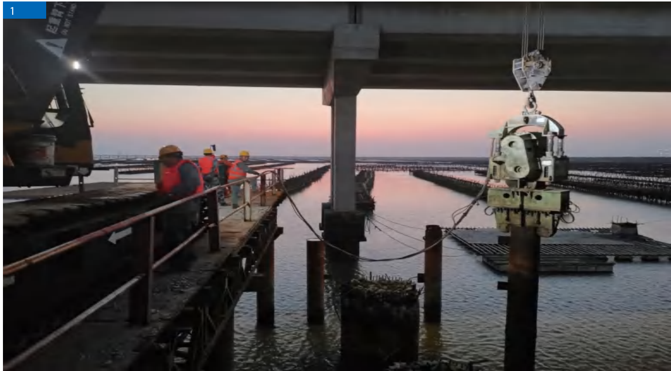
DZJ-90 1 湛玉高速一工区东海岛大桥 Donghaidao Bridge,Yuzhan Expressway 1st Work Area 使用单位：中交一航局 User: CCCC-First Harbor Eng Co.,Ltd 施工情况：拔630管，长24m Construction situation: Extract 630 pipe pile,the length is 24m 入土深度：20m Depth of penetration: 20m
